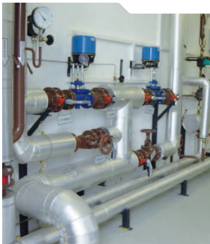
Delivery of heating water pipelines and controls
