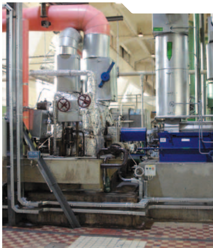
PC 850 driving turbine with a feed pump
