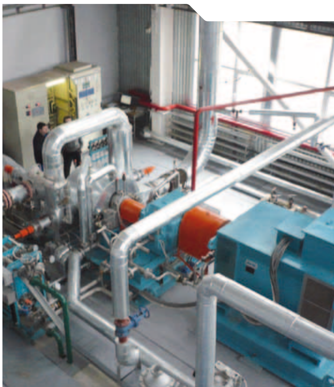
TG steam back-pressure turbine in commissioning
