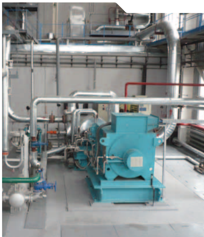
TG steam back-pressure turbine designed to drive a generator
